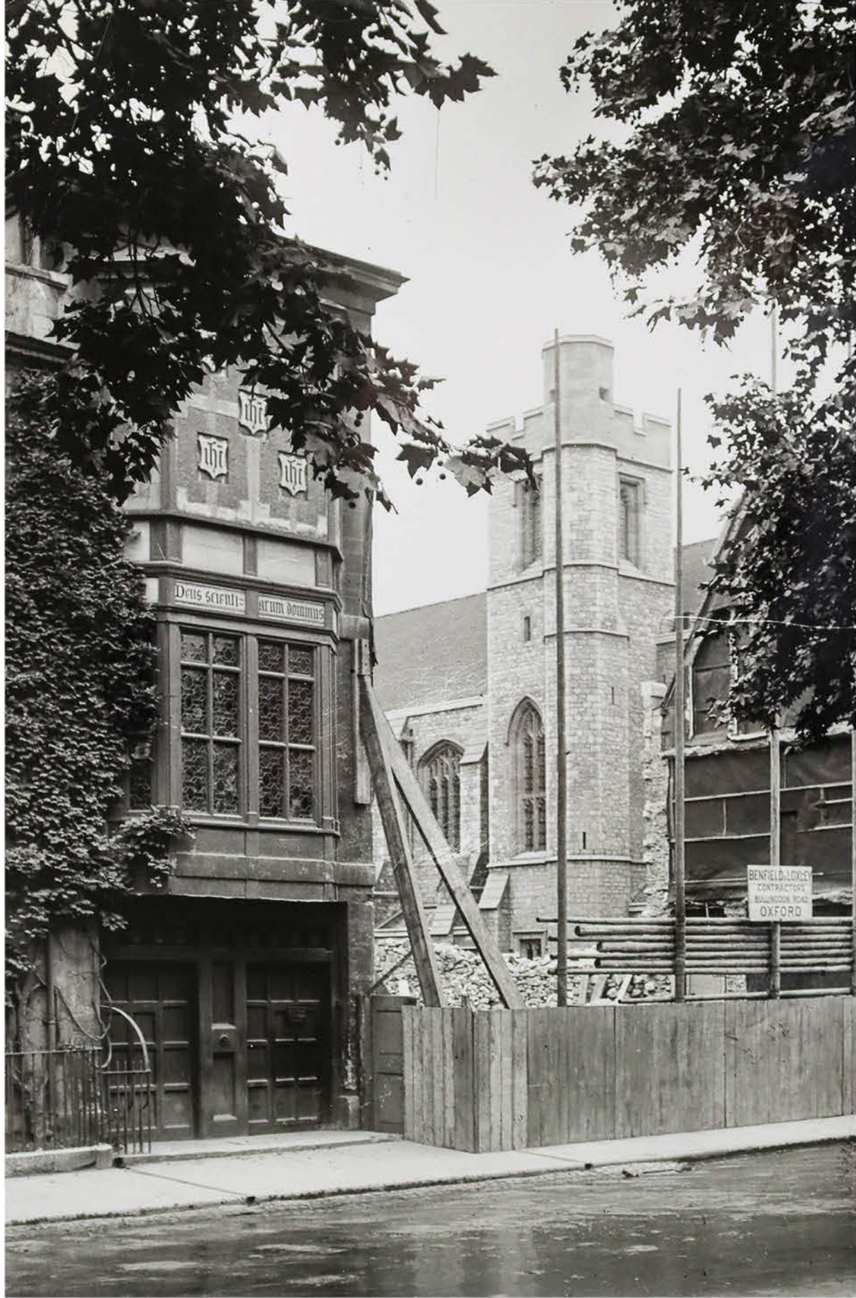
ABOVE: Pusey House under construction, ca. 1914
