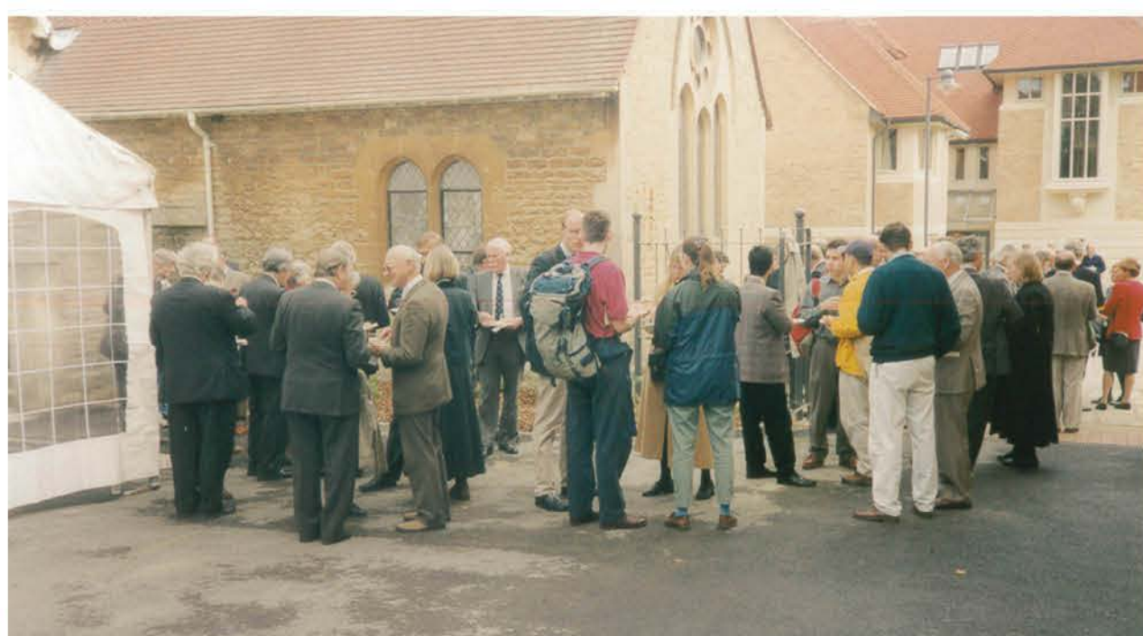
ABOVE: Replacing the hut with the Annexe 1995-96
