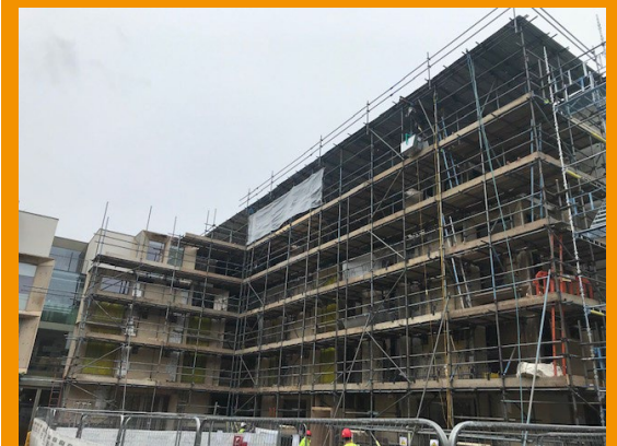
Courtyard access scaffolding
