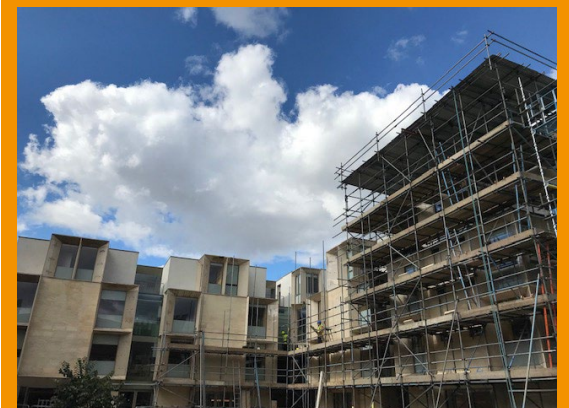
Courtyard access scaffolding
